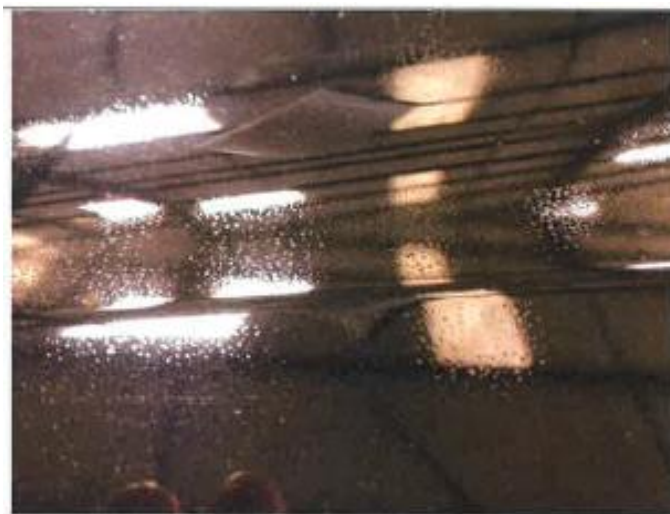
Close up of hood showing blistering
